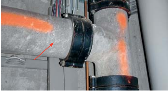
Tubo in fibrocemento
